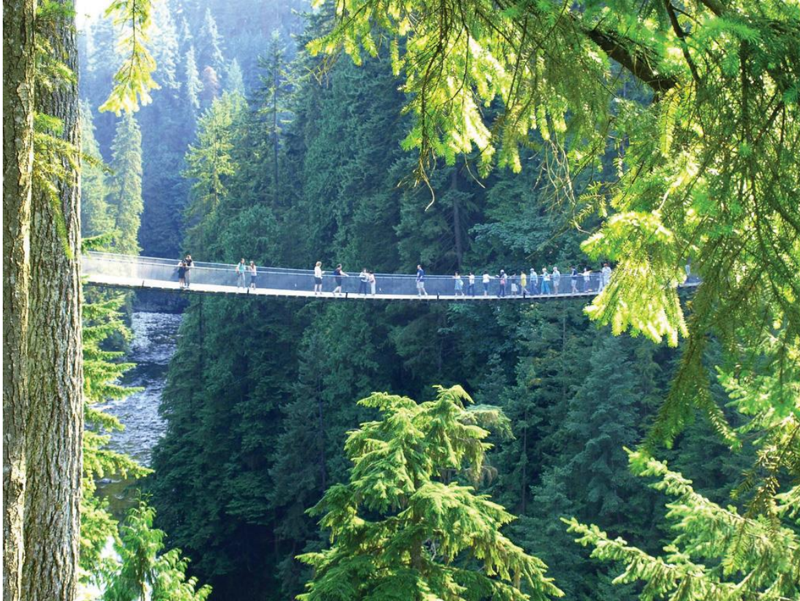
Figure 7.8 Capilano River Bridge
